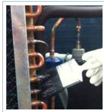
Corrosion inhibiting coating applied throughout the unit
